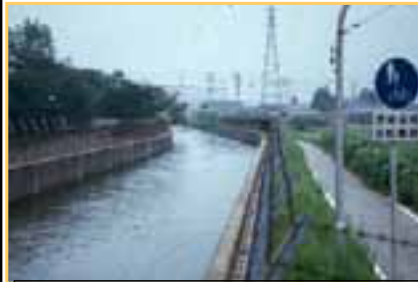
Modernized: Made of concrete and guarded by fence to prevent children from jumping into the canal
